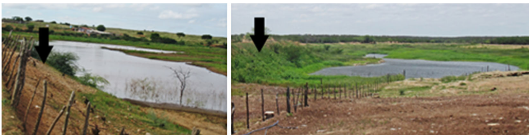
Fig. 9 Water tanks ( Barreiro ), the arrows indicate the earth bus that allows the accumulation of water. Record in the surroundings of the Poçoões community, in the Paraíba River basin, semiarid region of Brazil
